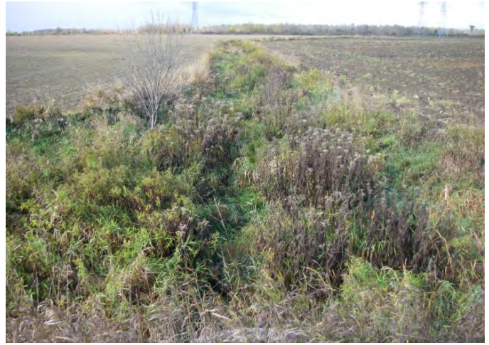
Photo 26: Station 17-1 – Gajtani Drainage Works (Fall 2012) - Facing upstream (west) from Sideroad 27 & 28, showing channel overview and adjacent agricultural fields.
