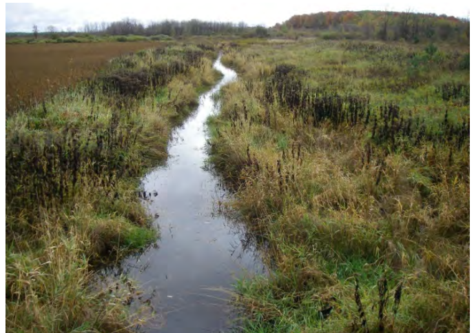
Photo 12: Station 6-2 – No. 21 Drainage Works (Fall 2012) - Facing downstream (east) south of 20th Sideroad, showing channel overview and adjacent fields.
