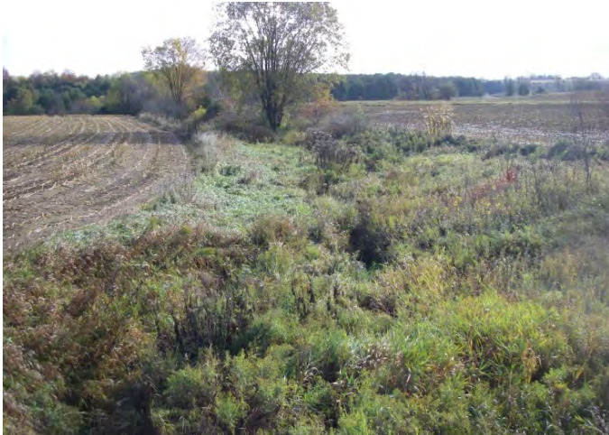
Photo 27: Station 17-1 – Gajtani Drainage Works (Fall 2012) - Facing downstream (east) from Sideroad 27 & 28, showing channel overview and adjacent agricultural fields.
