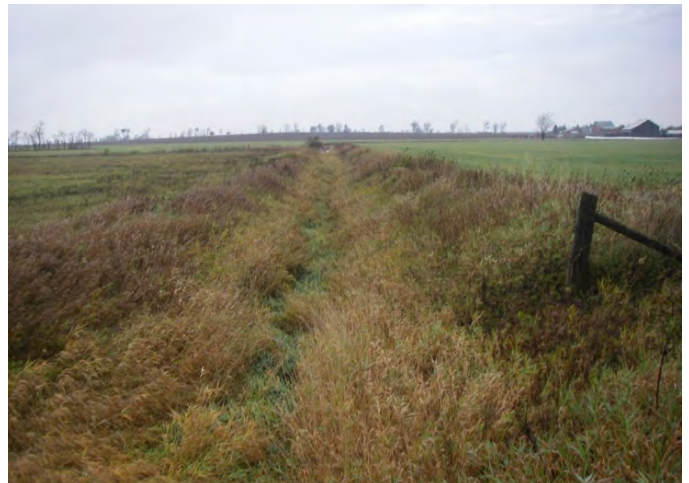
Photo 42: Station 1-3 – No. 2 Drainage Works (Fall 2012) - Facing downstream (north) from Concession 2 & 3, showing channel overview.
