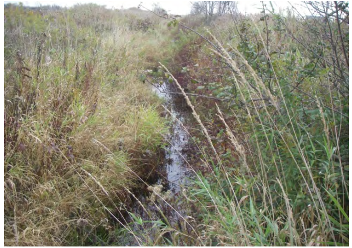
Photo 44: Station 1-1 – No. 2 Drainage Works (Fall 2012) - Facing downstream (east) from Concession 2 & 3, showing channel overview and surrounding riparian vegetation.
