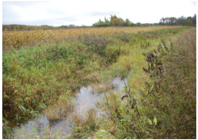
Photo 8: Station 6-1 – No. 21 Drainage (Fall 2012) - Facing upstream (west) from Concession 8 & 9, showing channel overview.
