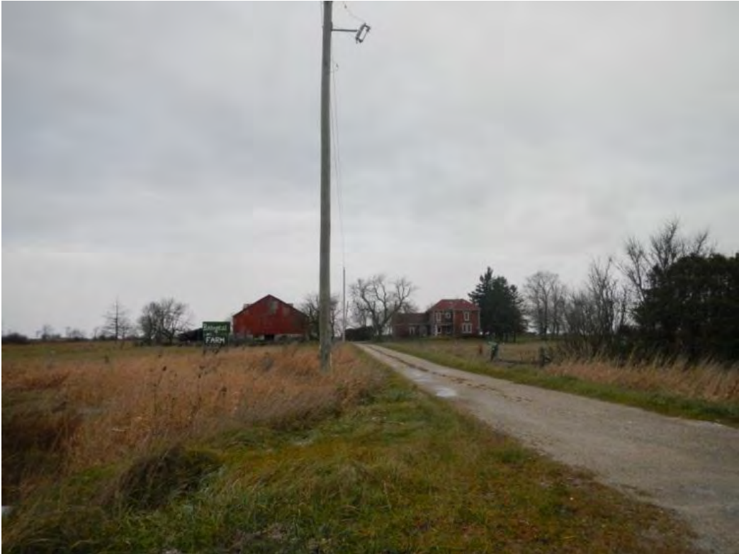
Photo 30: Farm complex, 202289 County Road 109 (Map 9)
