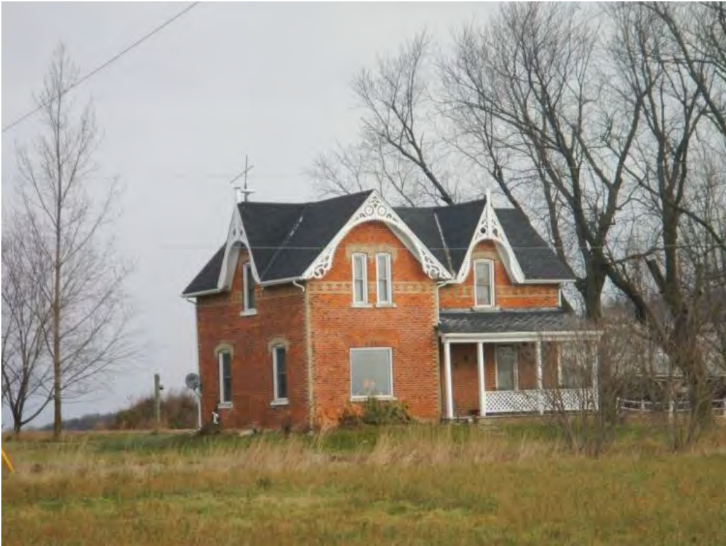
Photo 52: Front elevation, 113339 Sideroad 27/28 (Map 9)
