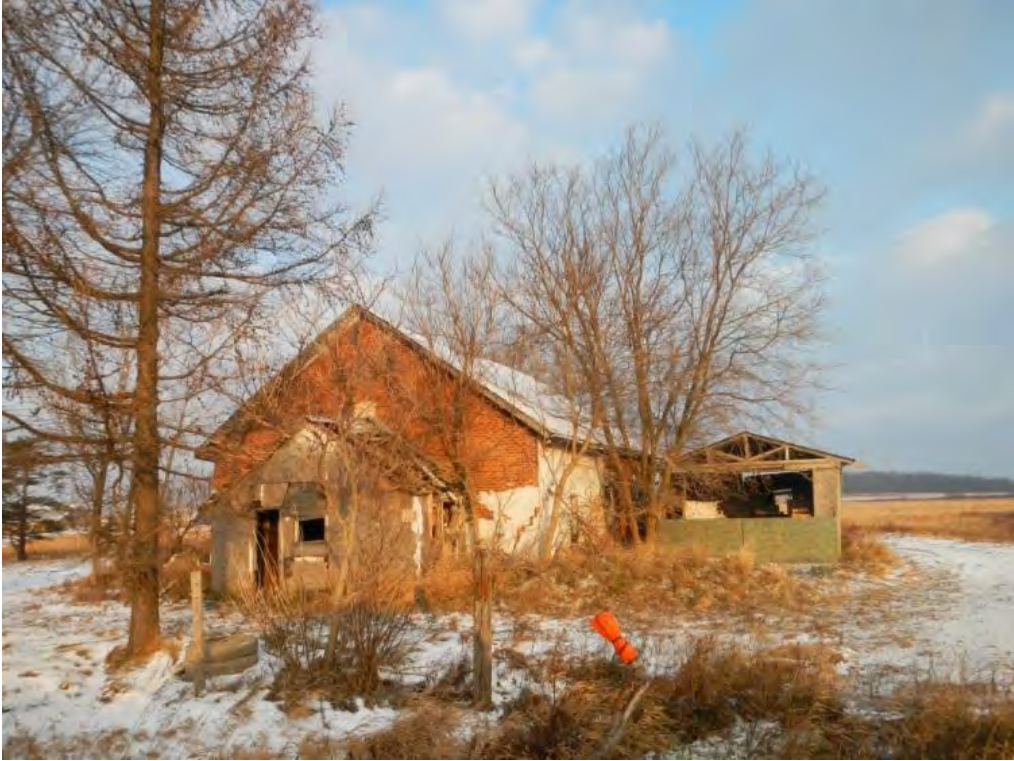
Photo 105: Vacant building on Highway 89 (Map 1)
