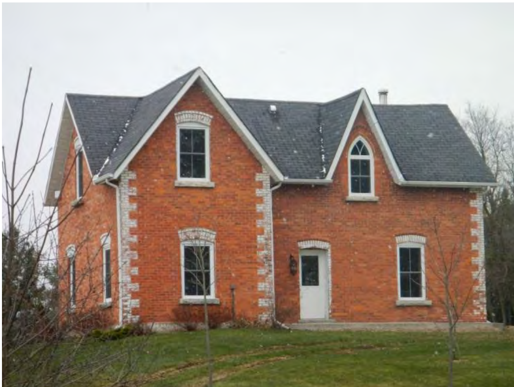
Photo 68: Front elevation, 114520 Sideroad 27/28 (Map 5, inset 2)
