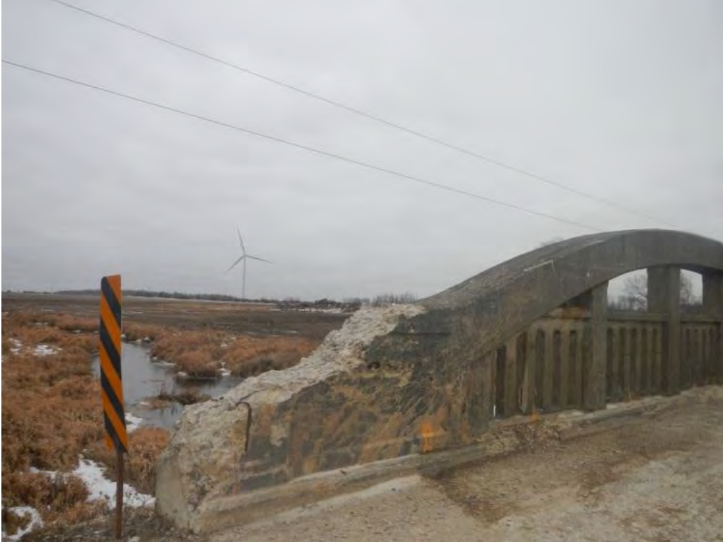
Photo 269: Bridge along Sideroad 27/28, south of Highway 89 (Map 2)
