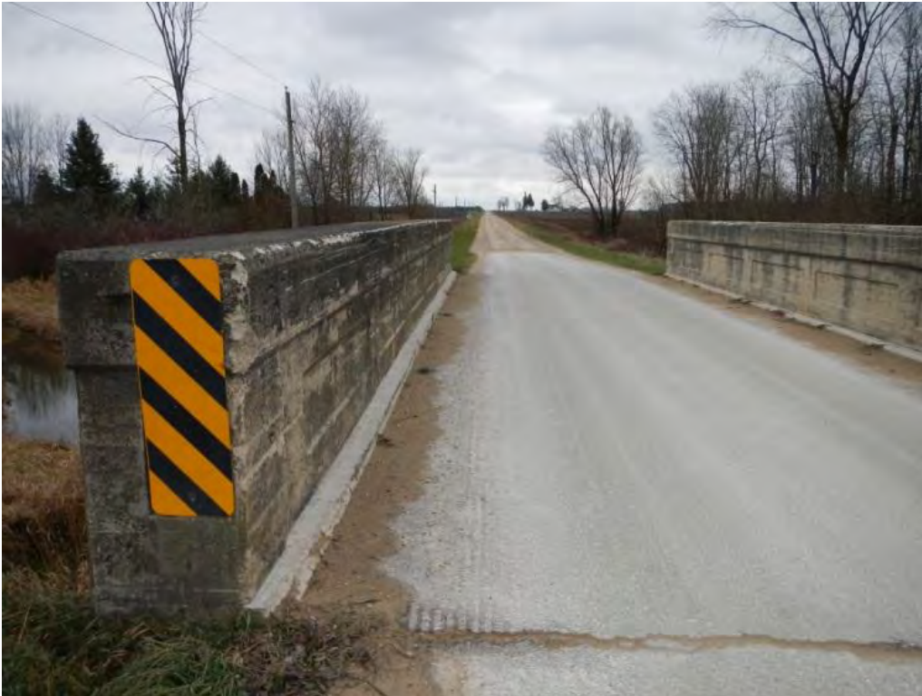
Photo 74: Bridge on Sideroad 24/25 (Map 4)
