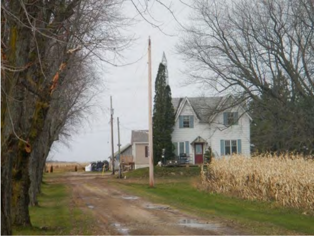
Photo 51: Front elevation, 113122 Sideroad 27/28 (Map 9)
