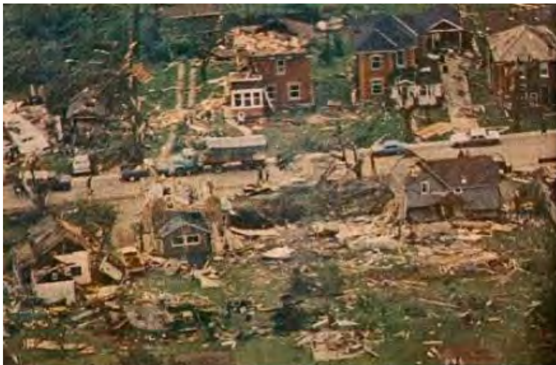
Plate 1: Photograph of Amaranth Street, Grand Valley following 1985 tornado (Bruineman, 2010).
