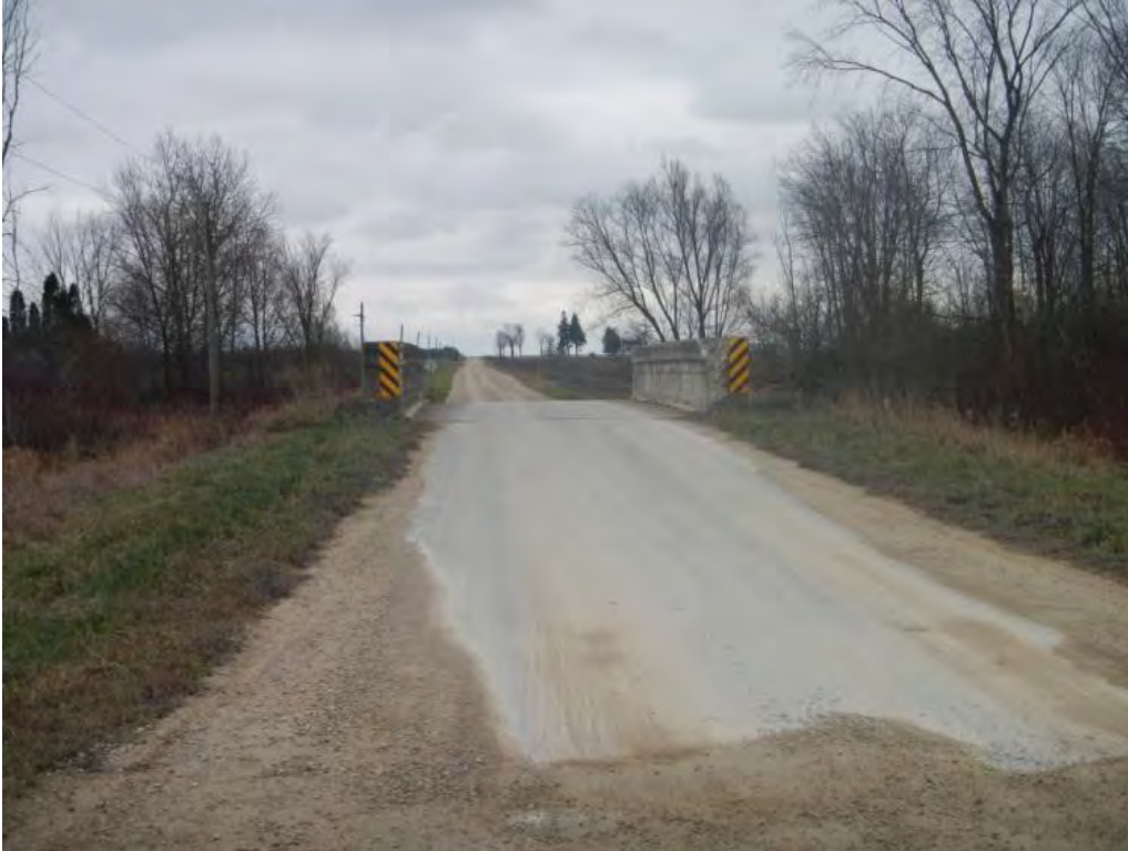
Photo 73: Bridge on Sideroad 24/25 (Map 4)
