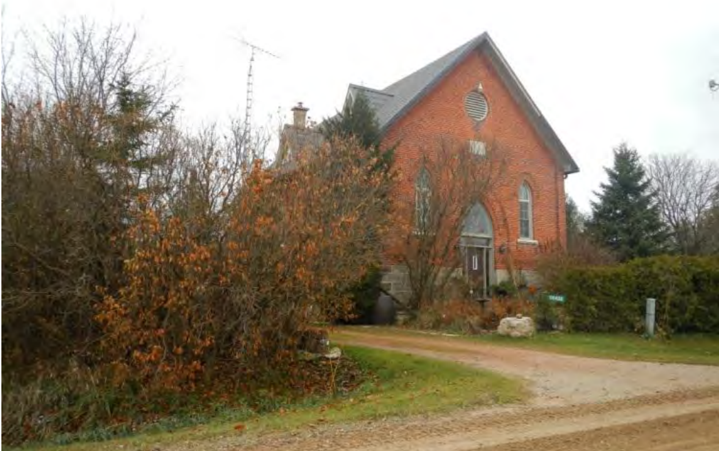
Photo 64: Front elevation, 114408 Sideroad 27/28 (Map 5)
