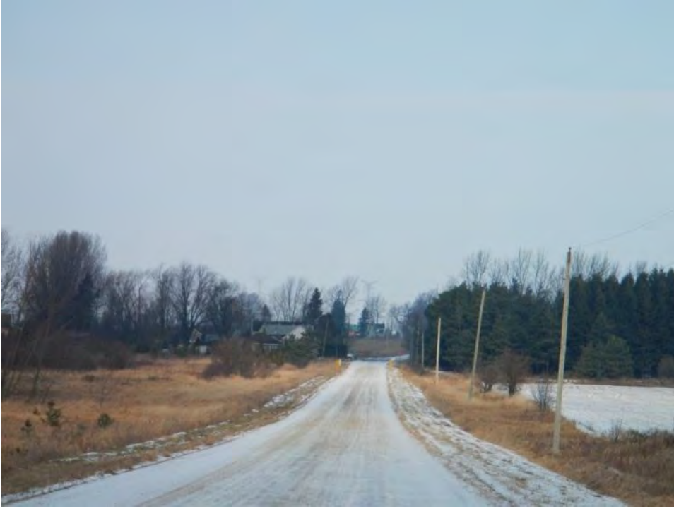
Photo 130: Monticello, streetscape, Sideroad 21/22 (Map 4)
