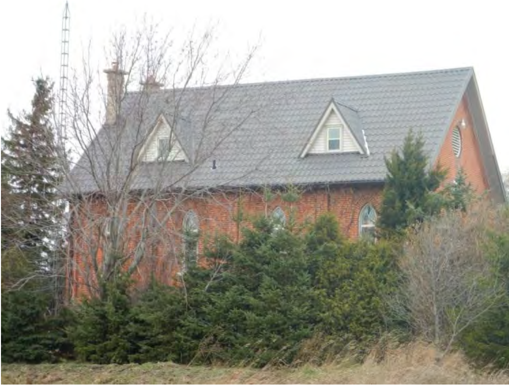
Photo 63: 114408 Sideroad 27/28, south elevation (Map 5)
