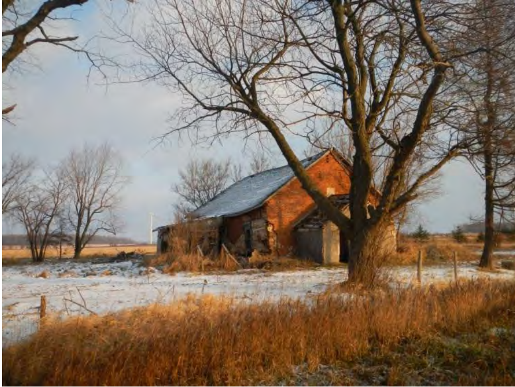
Photo 107: Vacant building on Highway 89 (Map 1)
