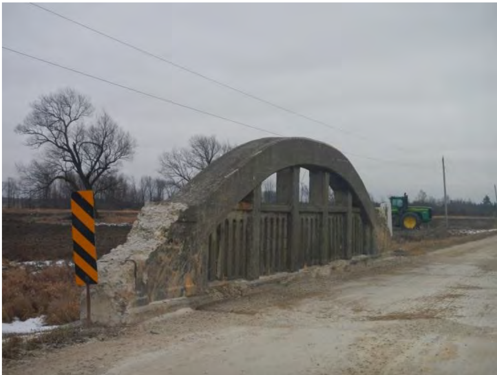
Photo 268: Bridge along Sideroad 27/28, south of Highway 89 (Map 2)
