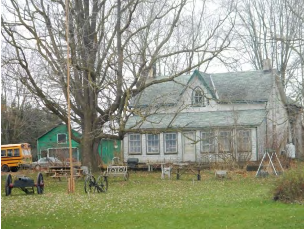
Photo 59: Front elevation, 114242 Sideroad 27/28 (Map 6)
