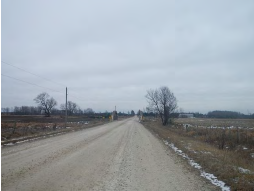
Photo 267: Bridge along Sideroad 27/28, south of Highway 89 (Map 2)
